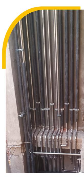
Further, Primegold Pipes & Fittings have lower friction as compared to cement lined or corroded carbon steel pipes ensuring less loss of water pressure along the pipeline. This provides an opportunity to diminish the internal diameter of the pipe and save capital cost. This is also a reason for a lower adhesion of deposits as well as lower bacteria colonization. It is also tolerant to high flow rates.
